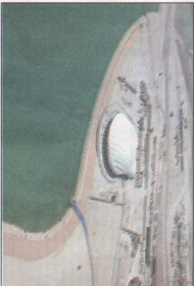
Work in progress at the site of The Pearl-Qatar project
